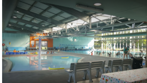
Yarra Aquatic Centre, Shire of Yarra Valley
